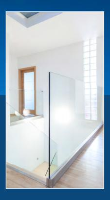
POSIglaze is extremely versatile, achieving force load resistance from 0.36kN to 1.50kN, making it suitable for domestic to light commercial installations.
